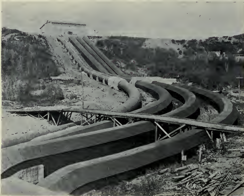
Forebay and Penstocks—No. 4, to left, 740 ft. long, 11 ft. diameter.
